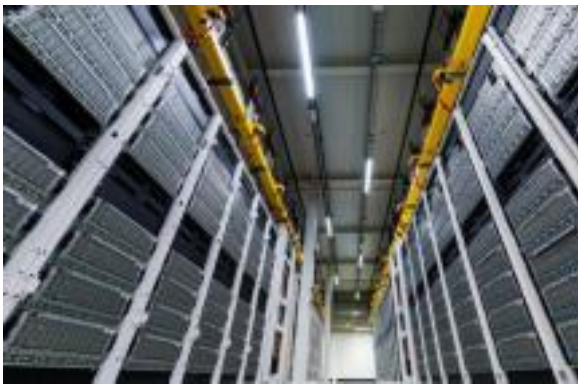
Fig 1. Data center Site (PHX region)
